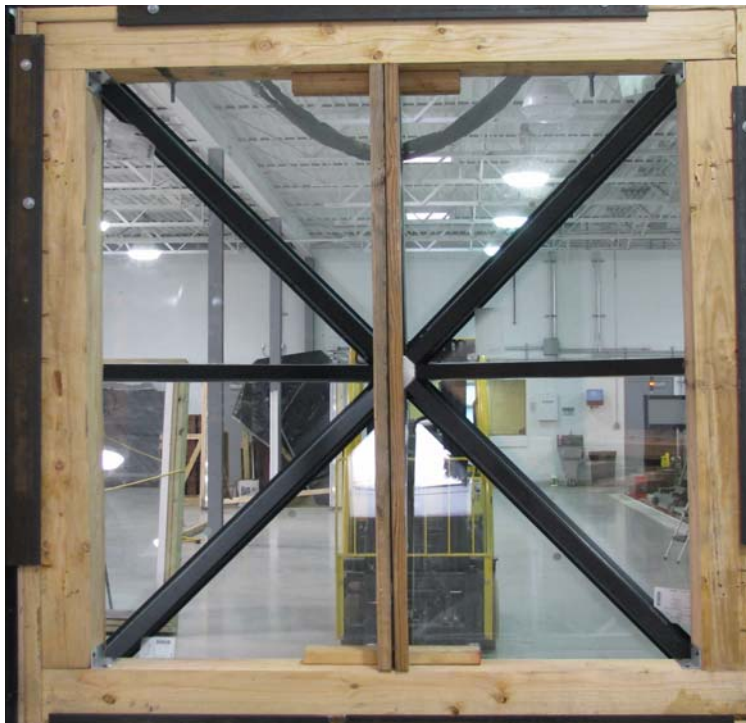
Photo No. 5 Post-test Specimen #2, Interior
